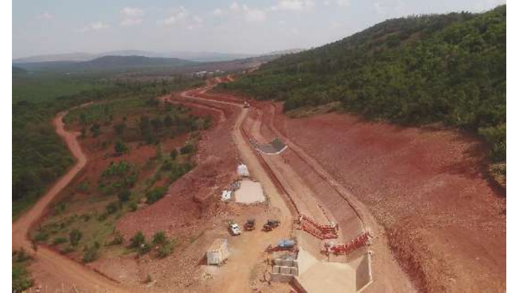
Excavation and backfill pool1
