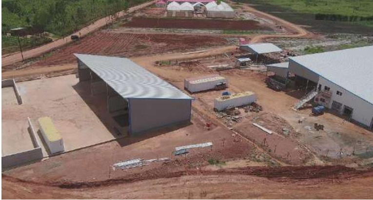
Demo Dairy at completion stage
